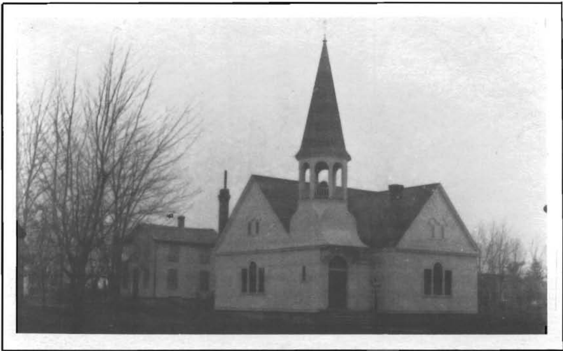
"Little" Presbyterian Church, altered to the former Alta Wilson home. This is located at the corner of Church & Church & Adams, 108 S. Adams.
