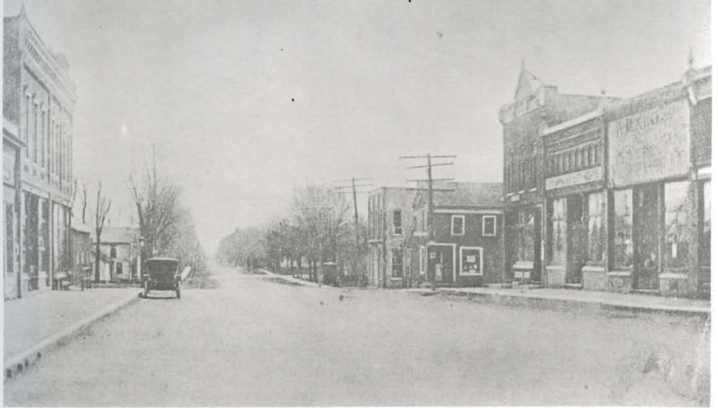
Main Street looking south in the early 1900's.
