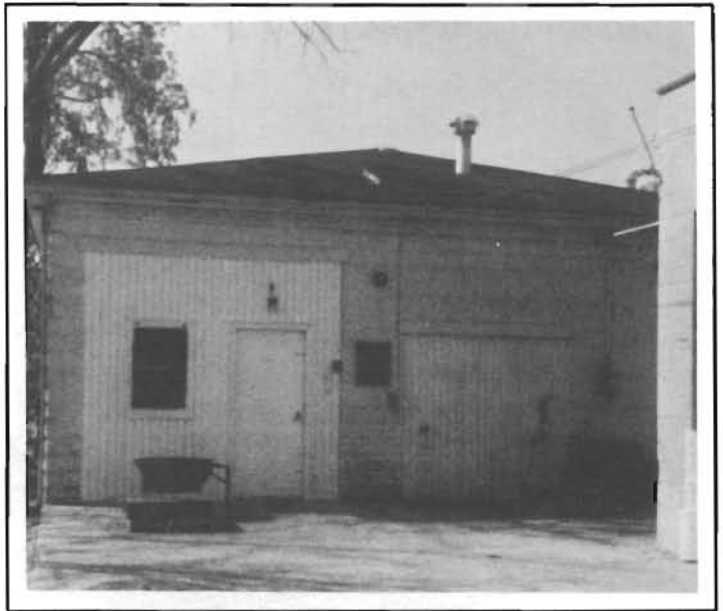
Water Plant - 106 E. Sigler behind the Town Hall.
