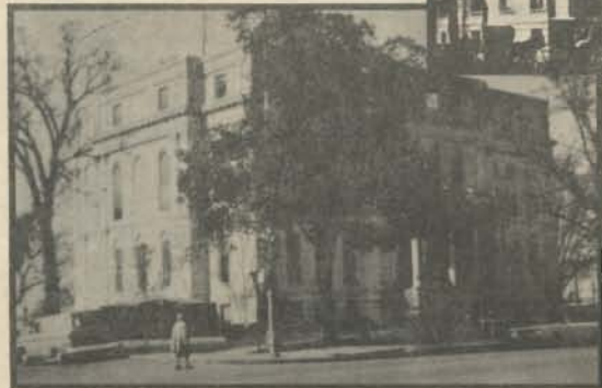
At left: Restored Courthouse in recent years.
