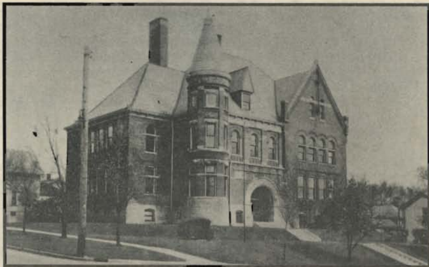
Columbia School southeast corner Indiana & Locust. Dedicated Jan, 13, 1893. Today's site for Columbia Apartments.
