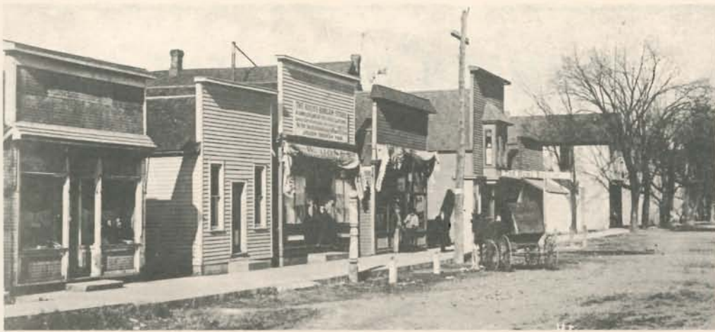
WEST SIDE OF MAIN STREET, LOOKING NORTH
