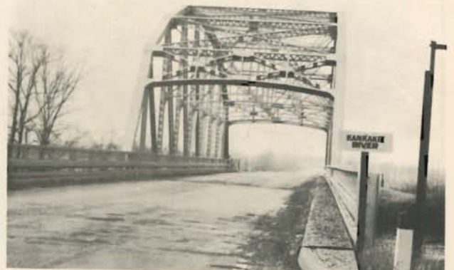
River Bridge on Highway 49
