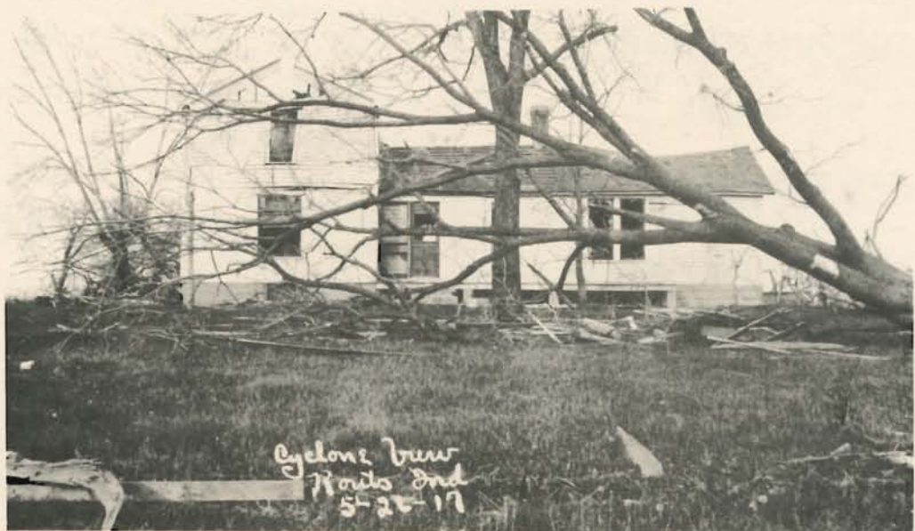
Henry Glissman home after the tornado (now the home of Mr. and Mrs. Ralph Riley)
