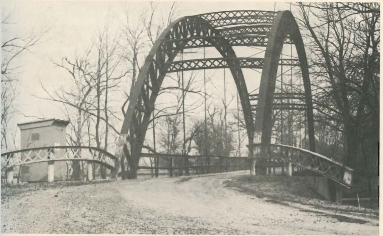
Dunn's Bridge over the Kankakee River. (Built from part of the Ferris Wheel used in World's Fair in 1893).
