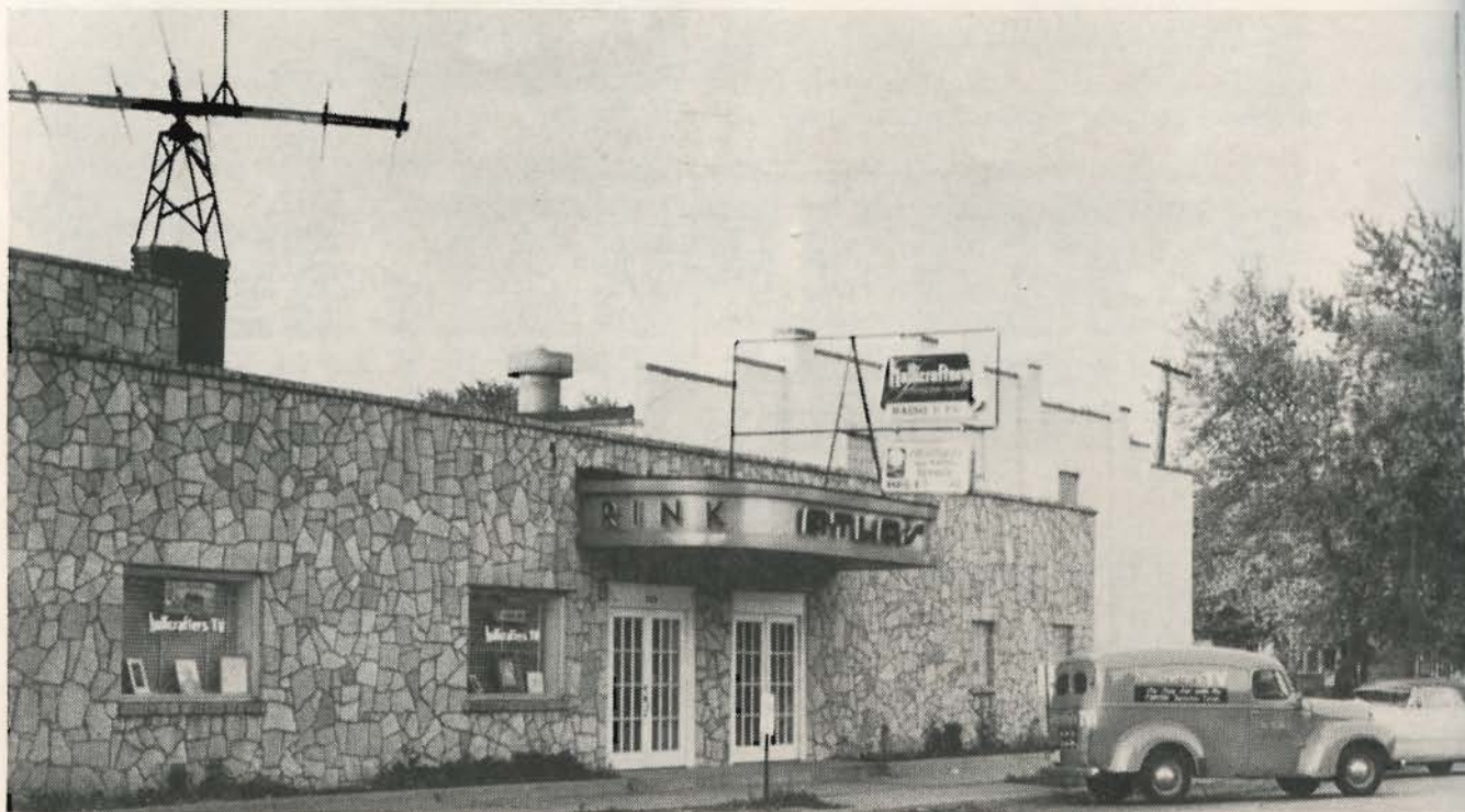
Chesterton's Only Apartment Building, Built 1946-1948.
